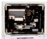
**HEATING/FURNACE** - Thermostat, thermocouple, main gas valve, igniter, burner assembly, blower motor, fittings, connections, and the PC board.
